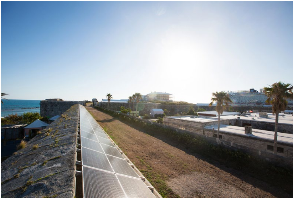
Solar panels were installed on the Grade 1 listed rampart wall of the Bermuda National Museum, in a discreet location away from Commissioner's House.
