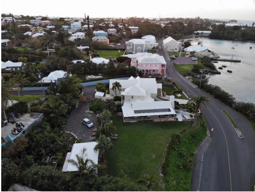
Solar panels were installed on the flat roof of the new west facing porch extension on Grade 2 listed Loyalty Inn.
